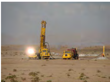
LEFT: Drilling in progress on the central Namib gravel plains. This is an archaeologically sensitive surface and detailed survey should precede drilling.
